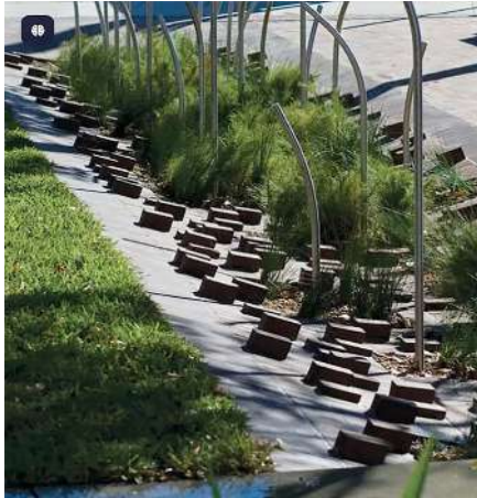
Figure 5. Brick Swale as a drainage system
