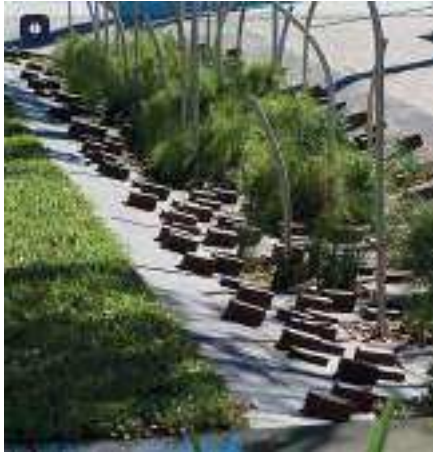
Figure 5. Brick Swale as a drainage system
